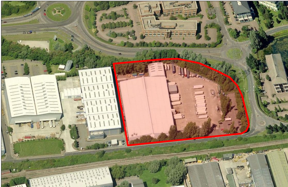
SITE AERIAL VIEW (Site area highlighted in red)
