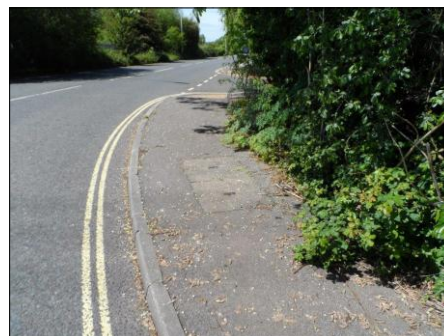
PHOTOGRAPH 2 EXISTING BT CHAMBER IN FOOTWAY ON BRUNEL ROAD TO EAST OF ENTRANCE
