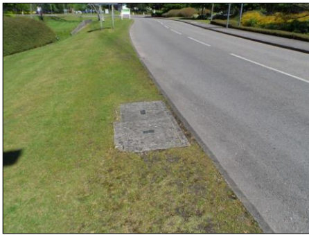
PHOTOGRAPH 4 EXISTING VODAFONE CHAMBER IN VERGE ON WEST SIDE OF WATERSIDE DRIVE
